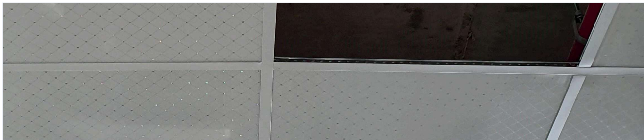
Cielo raso modular instalado
